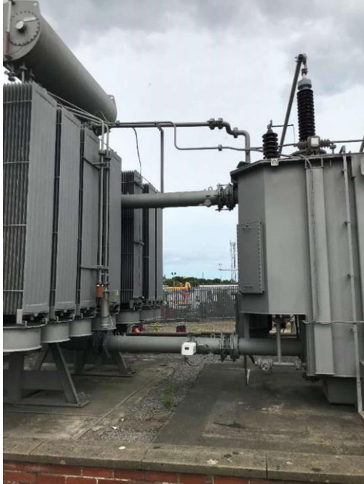
Figure 7: Photograph of the top and bottom oil lines of Scarborough Grid T2
