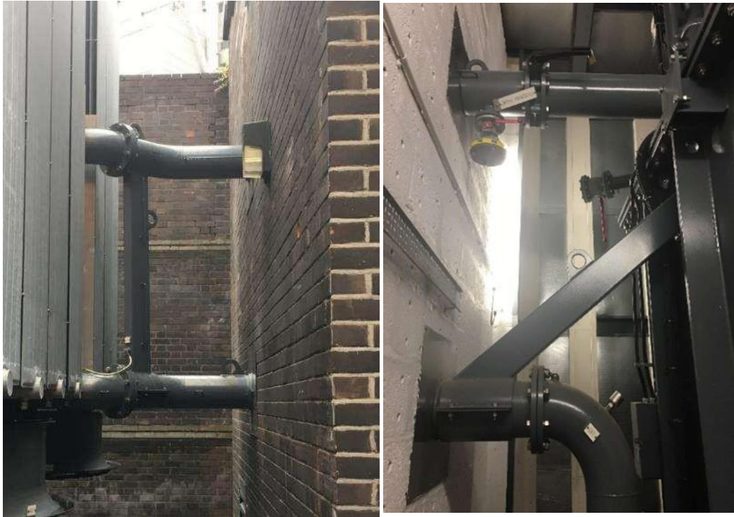
Figure 4: Photographs of the external (left) and internal (right) sections of the transformer top and bottom oil lines at the Barrack Road substation
