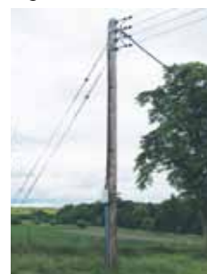
Figure 3: 400 V distribution line.
