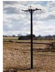
Figure 3: 400 V distribution line.
